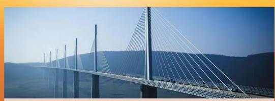
The addition of only 0.025% Niobium in the steel of the Millau Viaduct bridge reduced the weight of steel and concrete by 60% in the overall project.<sup>3</sup>
